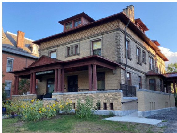
ADA accessibility ramp
